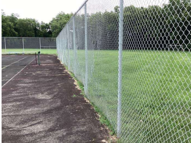
Chain link fence (note warped webbing)
