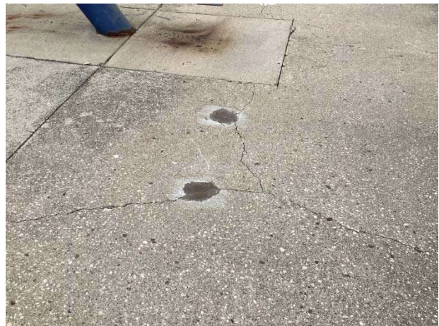
Concrete cracks
