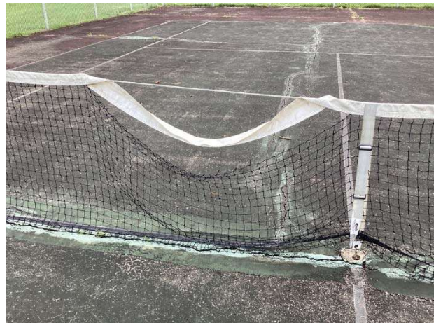
Pool house tennis court cracks (note net damage)
