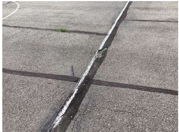
Pool house basketball court surface cracks and deterioration
