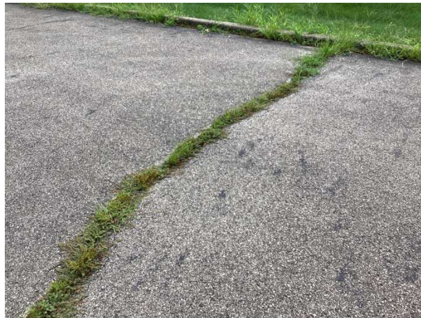
Willow Branch Drive pavement cracks (note organic growth)
