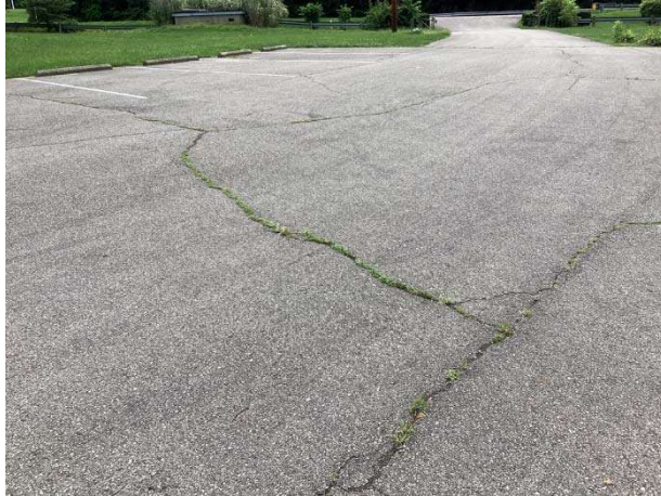
Willow Branch Drive pavement cracks
