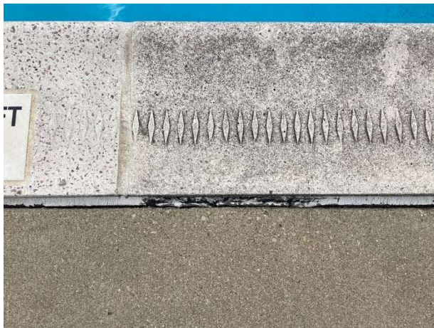
Joint sealant deterioration
