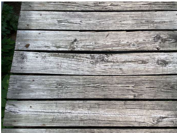
Weathered deck boards
