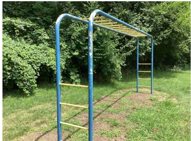
Forest Ridge Boulevard monkey bars (note finish deterioration)
