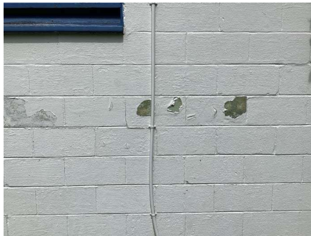
Paint finish deterioration
