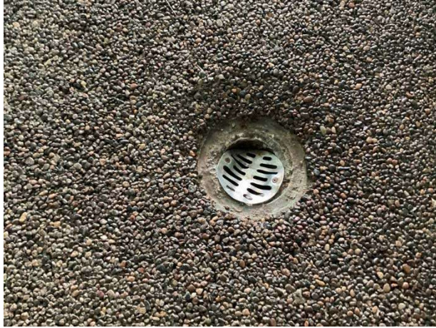
Displaced drain cover
