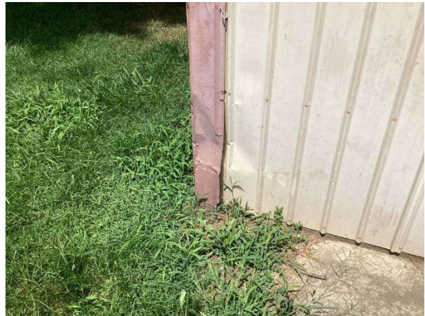
Siding damage
