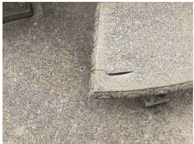
Concrete seat damage
