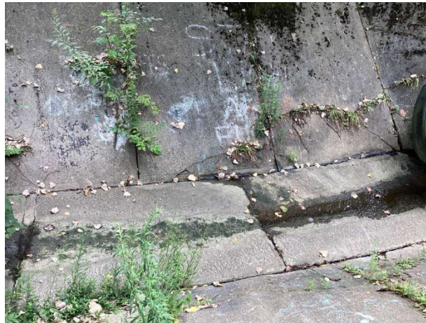
Culvert cracks
