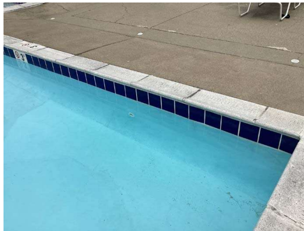
Pool plaster finish with tile perimeter
