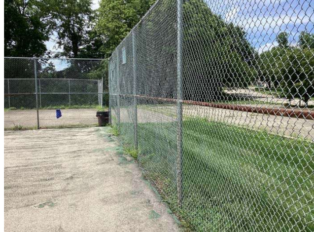
Willow Branch Drive fence (note warped webbing)
