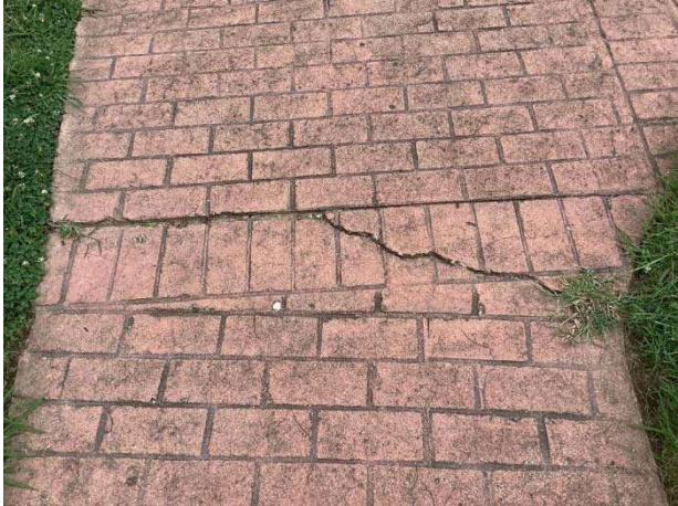
Stamped sidewalk cracks
