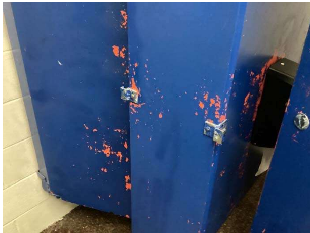
Partition finish deterioration
