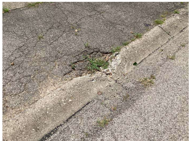
Concrete damage (Willow Branch Drive shown)
