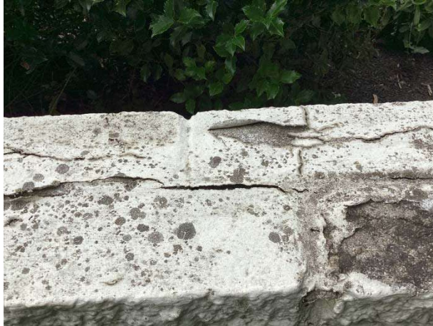
Paint finish deterioration
