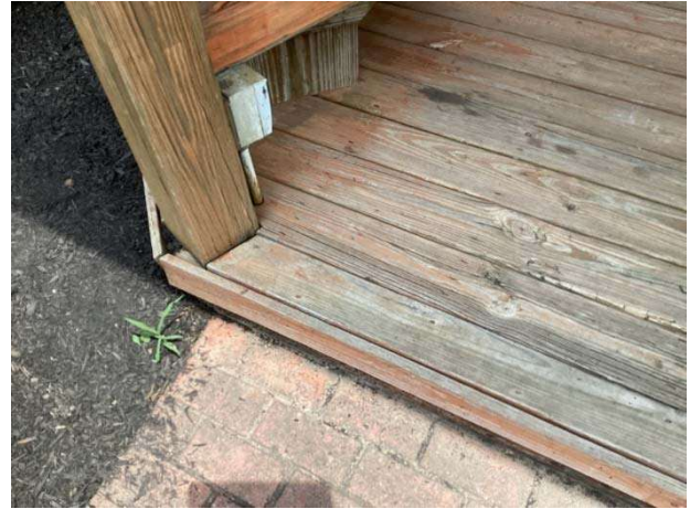
Gazebo decking (note finish deterioration)
