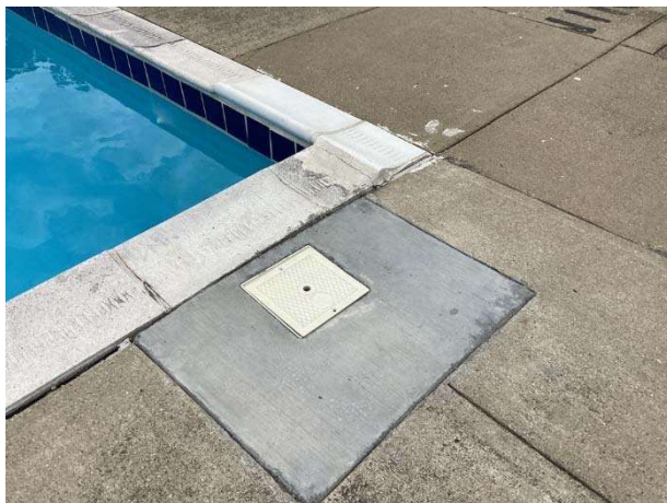
Concrete repair (note coping repair)
