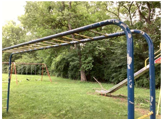
Meadowsweet Drive finish deterioration
