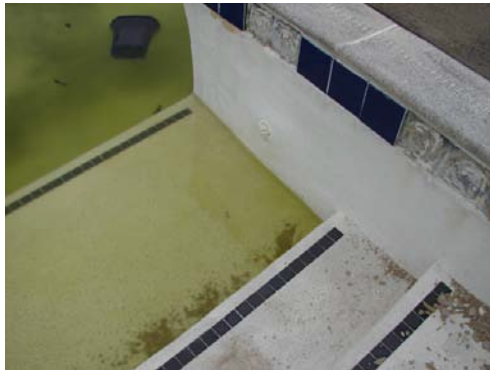
Water table tile needs replacement in diving pool.
