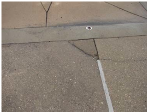
Cracking and pop-out areas of pool deck.
