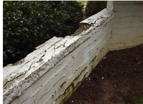
The extended brick walls of monument are deteriorating.
