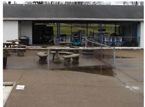
Due to the age of the pool deck many areas are sinking, causing standing water.
