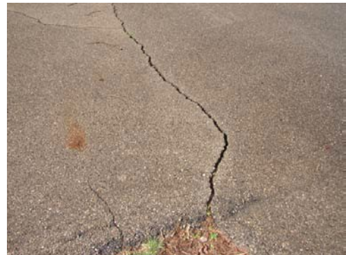
Cracking in asphalt pool parking area.
