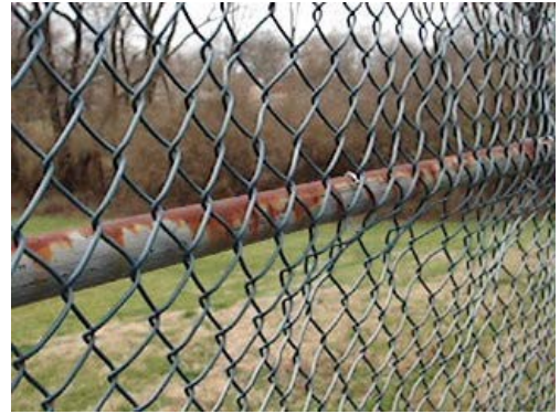
Chain link fencing in recreation area are rusting and bending in middle and bottoms.
