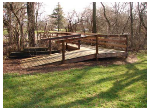
Wood bridge (7'w) with two wood rail and wood handrail.
