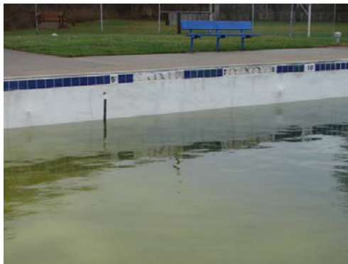
Diving pool missing water table tile, needs whitecoating and new concrete coping.
