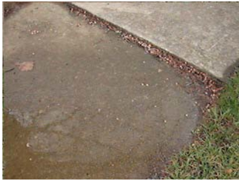
Settling of sidewalk along road causing a tripping hazard.
