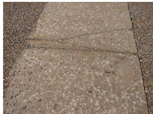
Cracked concrete sidewalk with salt deterioration at street in front of maintenance buildings.
