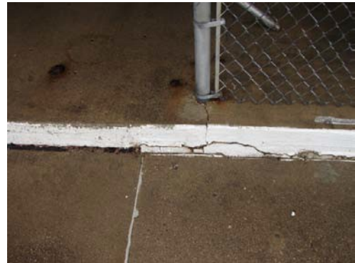
Transition between the pool deck and poolhouse picnic area is deteriorating and causes a severe tripping hazard.
