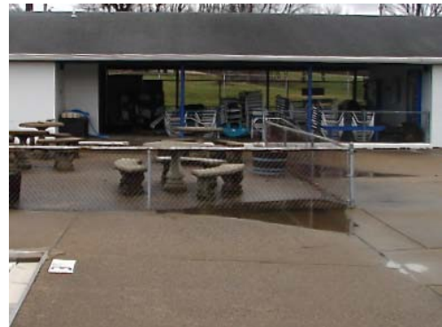
Concrete pool deck is sinking near racing pool and poolhouse.
