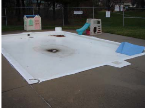
Wading pool with deteriorating coping. Pool has new filtering system.
