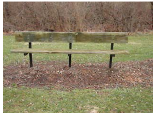
Typical bench at tot lot areas. Many boards are splintered, warped and not level.
