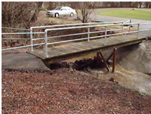
Wood bridge (4'w) with metal 2-bar railings over open storm water community creek.
