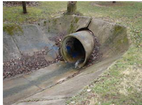
Typical storm bulkheads where community creek goes under the city roads. Assume the maintenance of creek bed in responsibility of association but not under the roads. These costs are included in Reserve Study.
