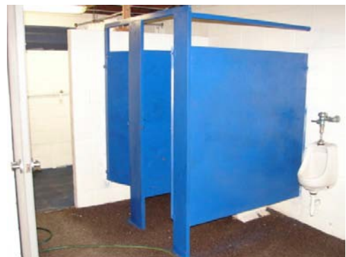
Typical wood partition stalls. Need of handicap upgrades in both restrooms.
