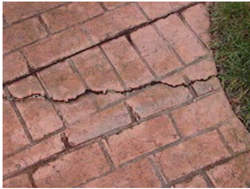
Stamped concrete brick with coloring sidewalk up to and around the gazebo has cracked in a few locations.
