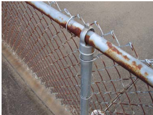
Lower fencing near wading pool showing rust.
