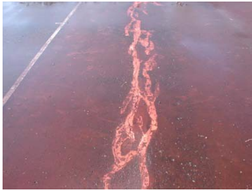
Typical cracks on tennis courts. Many cracks are on the playing areas. The colored surface coating has worn off.
