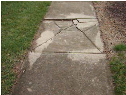
Concrete sidewalk between road and tot lot areas cracked and sinking.
