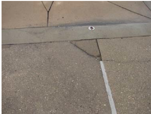
Concrete pool deck cracking in various areas.
