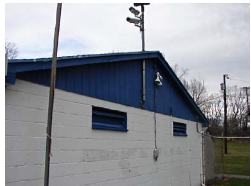
Wood T-111 siding in gables and screened/louver (8) openings in concrete block walls.
