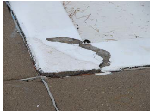
Coping deterioration around in wading pool.
